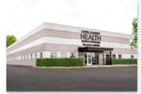
North Riverside Health Center
