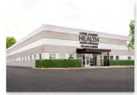
North Riverside Health Center
